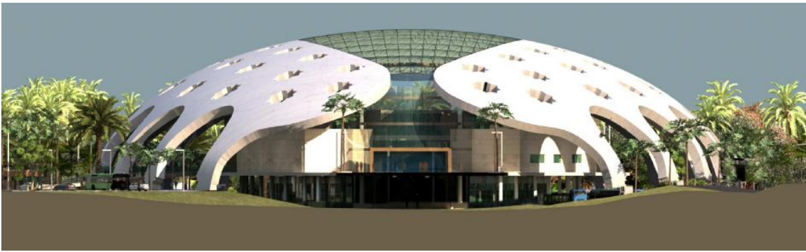
Argel's Intermodal Station, Algeria Engineering: SILGA S.L., Madrid Architecture: Tecnia Ingenieros
